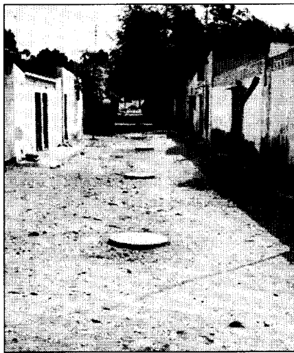
The sewer built by local people.
